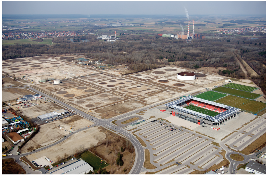
Copyright Bayernoil Raffineriegesellschaft mbH - Refinery Decommissioning April 2013
