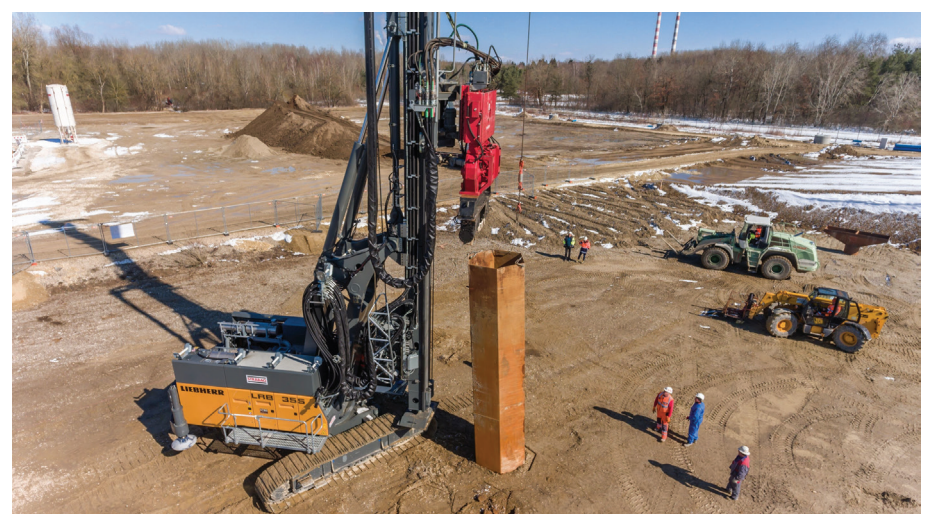
Copyright AUDI AG IN-Campus Pile driving for ground water capture
