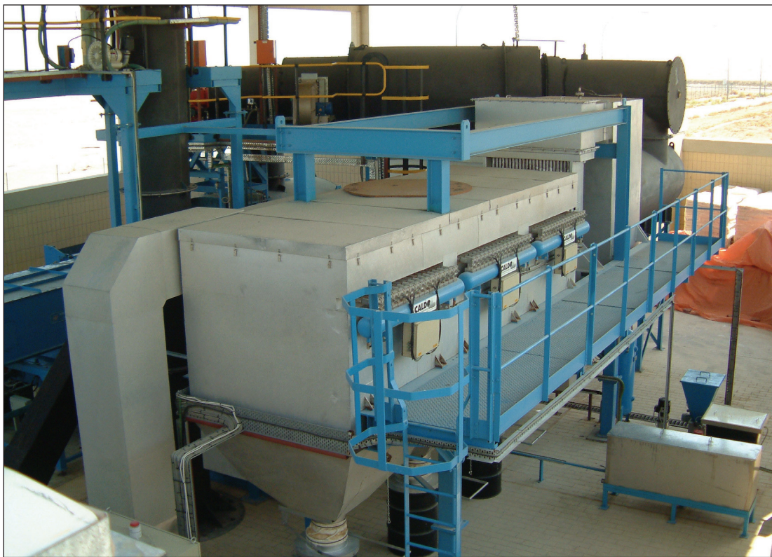
New hot gas filtration system for incinerators (Courtesy of Caldo Engineering)
