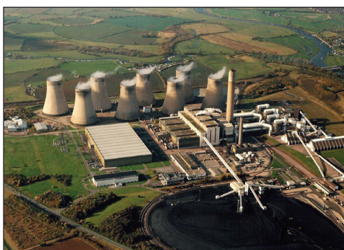
New filtration systems remove 98% of toxic flue gases. The real challenge is filtering out carbon dioxide. (Courtesy of EON, Radcliff-on-Soare)
