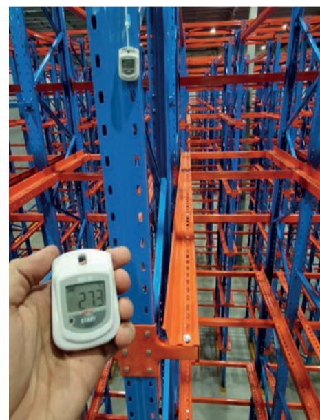
Multiple Ebro EBI 20 Data Loggers placed throughout a warehouse for continuous monitoring
