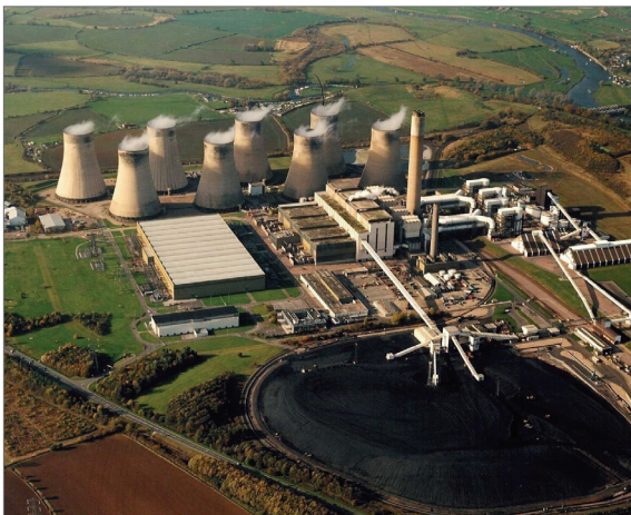
Figure 2. The EON Ratcliffe-on-Soare coal powered power station is on target to remove 98% of the sulphur dioxide from its flue gas.
