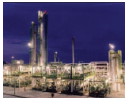
Figure 1. PEMEX, the largest refinery in Mexico
