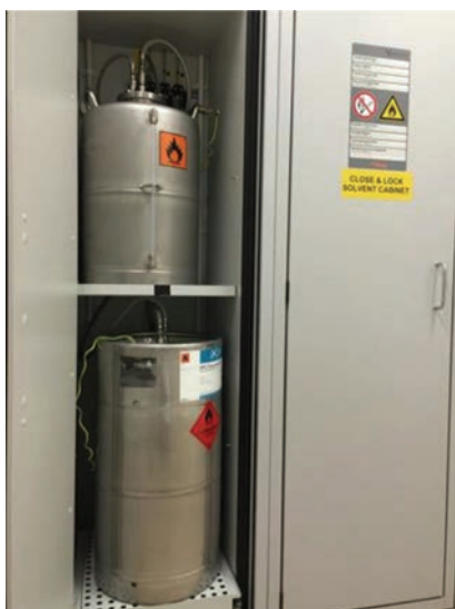
Figure 3: SFC co-solvent delivery solution with two 50 litre containers daisy-chained together. The container on the lower platform is replaced when empty, allowing solvent top-up without interrupting the purification campaign.
